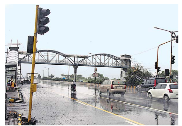
Many foot over bridges like this one on the Eastern Express Highway at Kanjurmarg will appear in the city
